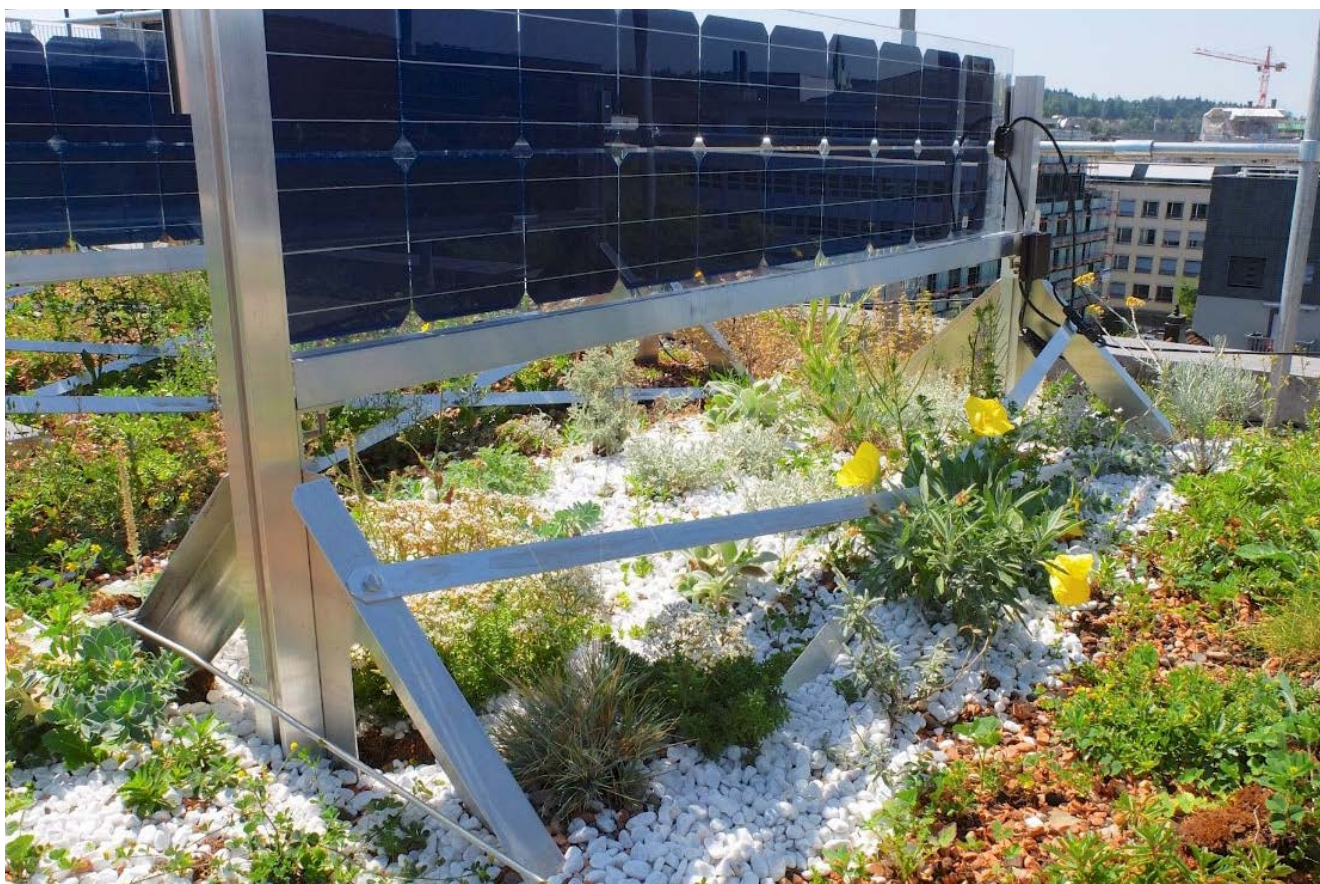
Figure 18: Installation test de la ZHAW, source: Solarspar
